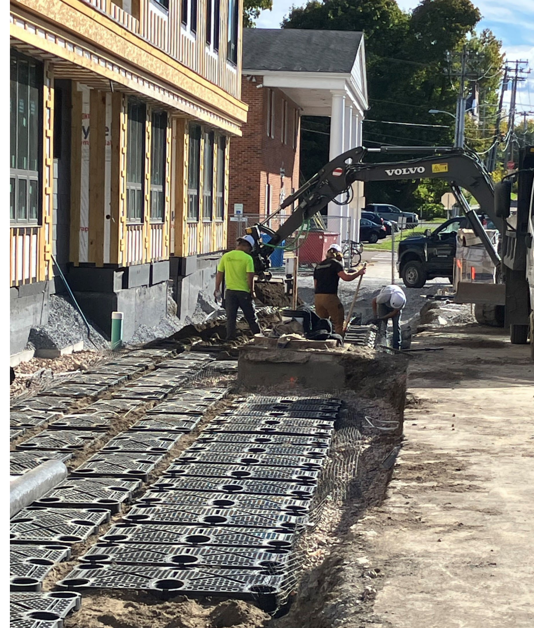
Urban Forestry Block Grant in action: Silva Cells installed at Winooski & Main (Burlington) to expand soil volume, manage stormwater, and ensure long-term canopy growth.
